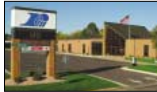
The expansion at Rice Lake more than doubled the size of the office.
